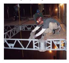
Safway electric hoists and modular staging systems fit through most boiler openings to help access areas for inspection, maintenance and repair.
