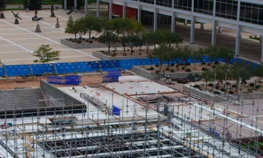
(ABOVE) Safway provided shoring in addition to scaffolding for the Air Force Academy project.
